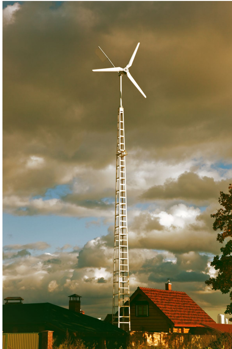
Figure 31. Small wind turbine for domestic use.
